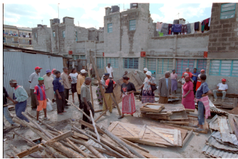
FIGURE 70. Taking down shacks to rebuild Kambi Moto.
