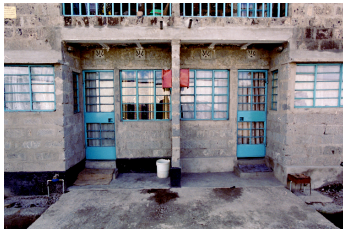
FIGURE 74. The entrance of the new houses in Kambi Moto.
