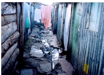
FIGURE 69. Corridor-like spaces in Kambi Moto.
