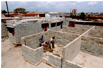
FIGURE 71. Construction in Kambi Moto.
