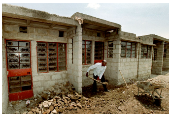
FIGURE 72. Construction in Kambi Moto.
